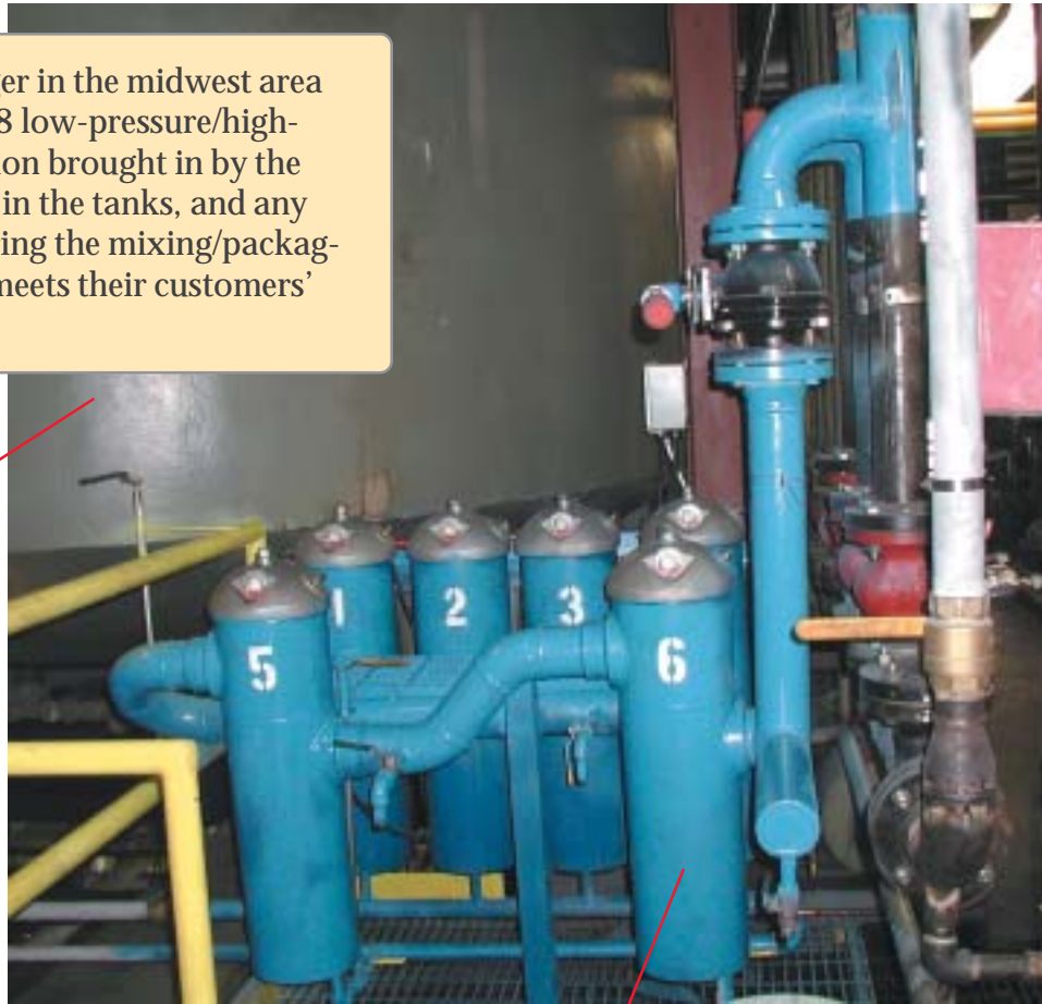
HFK08 Filters. 4 in parallel then 2 more in series -- for 3X filtration.
